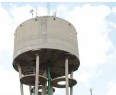
Elevated reservoir at the Optimum Coal Water Reclamation Plant.
