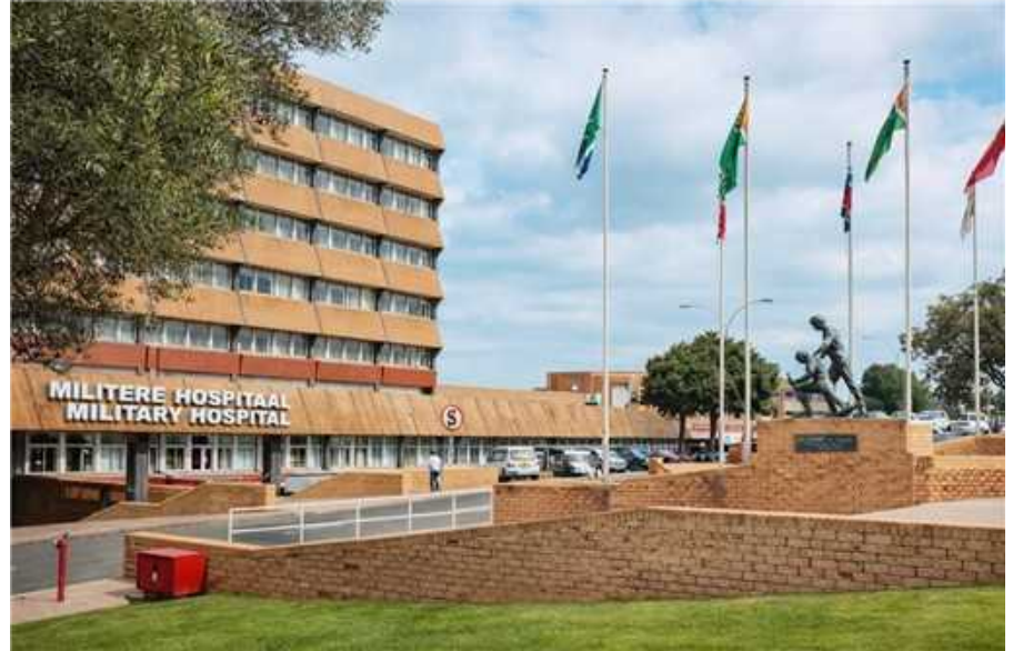
Main entrance of 1 Military Hospital at Thaba Tshwane, Centurion/Pretoria, Gauteng, South Africa.
